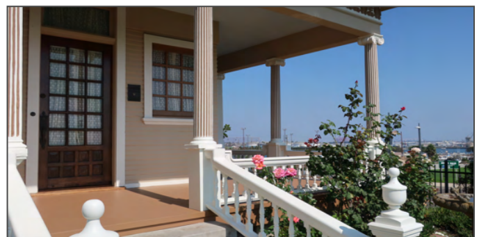
Freshly painted and restored porch area of the Muller House
