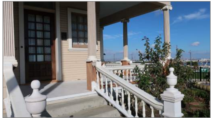
Restored banisters and railings, new finials and newel posts await more primer and top coats of paint.
